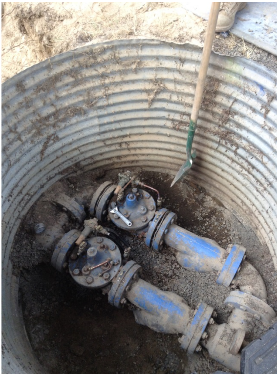
Figure 8 - Pressure Reducing Valves
