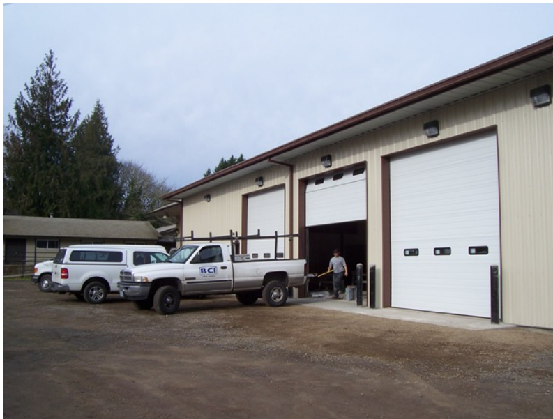
Warehouse constructed on North Umpqua Ranger District in 2011 – This proposed warehouse would be similar
