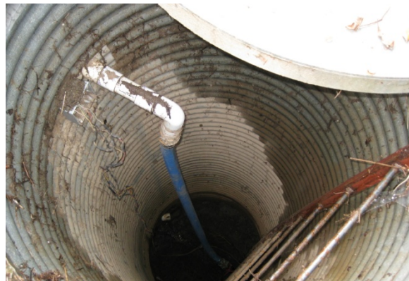
View into 42” CMP Vertical Pump Access Pit
