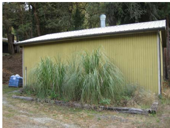
Water Treatment Plant Building
